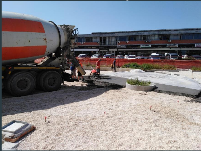
Base layer IN GRAVEL
